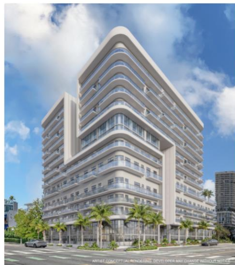
Robert Finvarb Companies recently started construction on NoBe Parc, a 15-story, mixed-use residential project that is part of a wave of new development coming to Miami Beach's North Beach neighborhood. (Courtesy of One World Properties)
